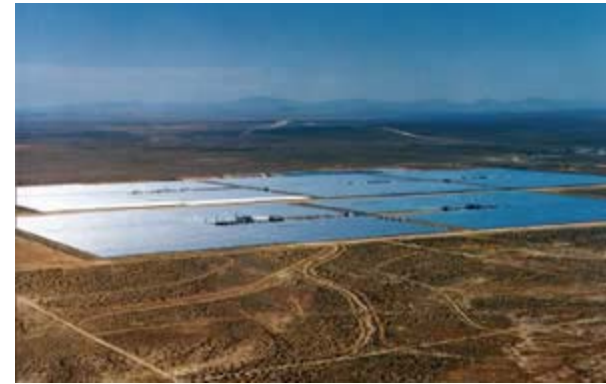
The world's largest solar power facility consists of five solar electric generating systems with a combined capacity of 150 MW, enough to power 150,000 homes.
