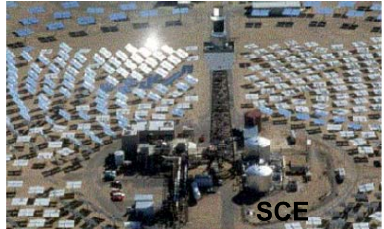
Solar Two Central Receiver (Power Tower)
