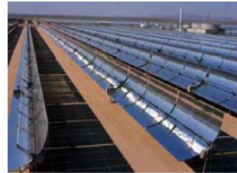
Central – Kramer Junction (CA) Solar Electric Generating Station
